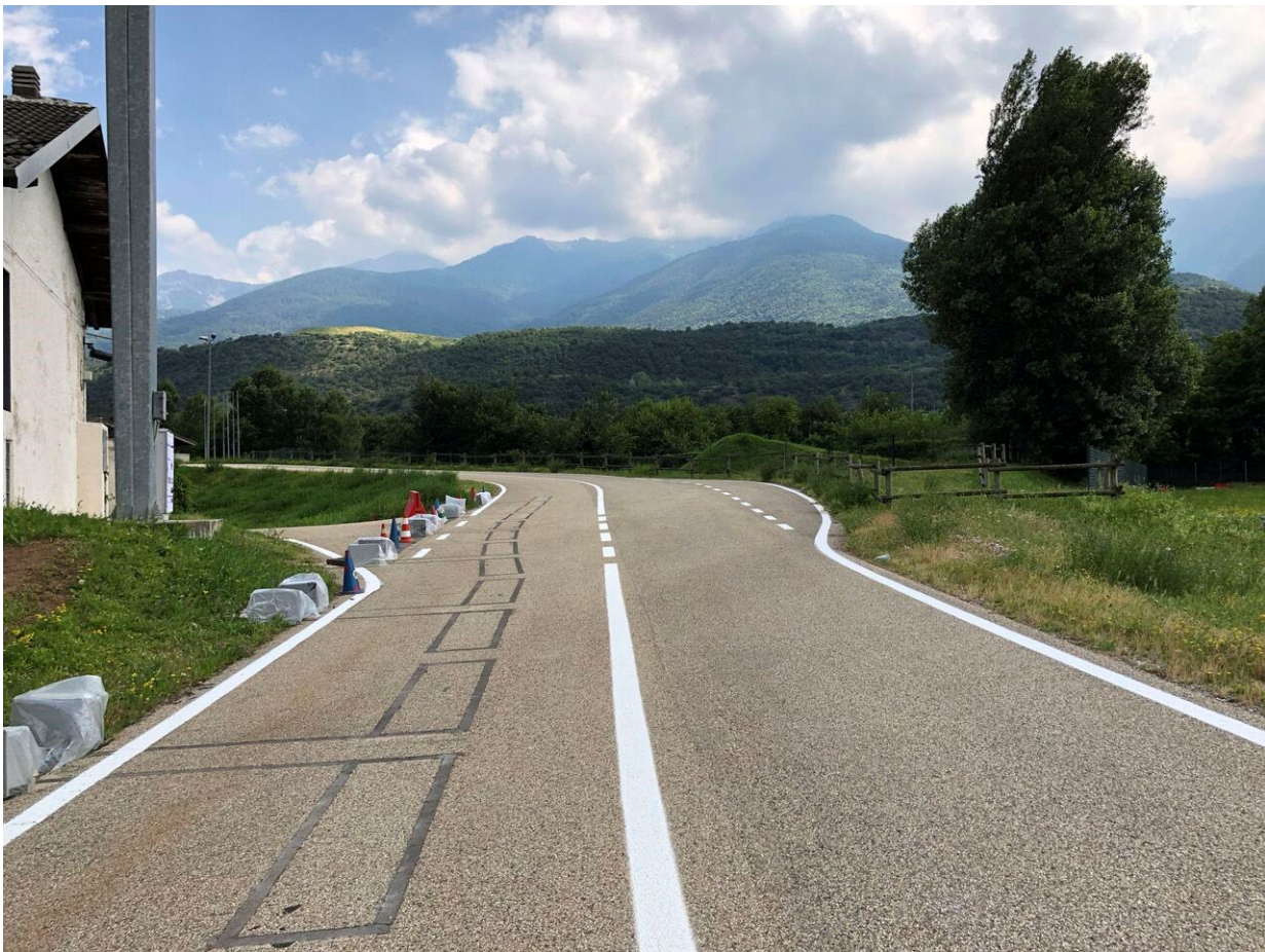
Figure 3. Politecnico di Torino and FABRIC's on-road WPT installation, Susa, Italy
